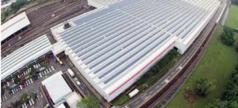
Solar panels installed on BSD rooftop
