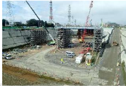
Kanagawa Prefecture Station (tentative name)
