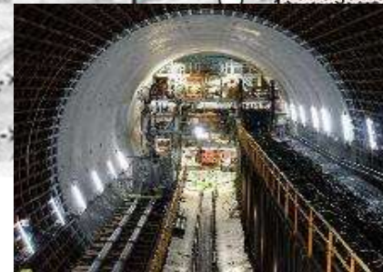
Metropolitan Area Tunnel No.1 (Kita-Shinagawa)
