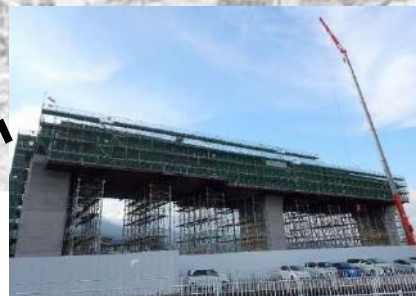
Viaduct in Yamanashi
