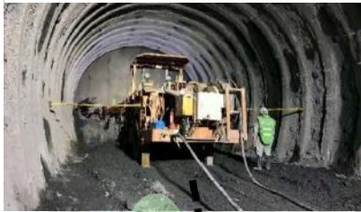
Southern Alps Tunnel (Yamanashi)
