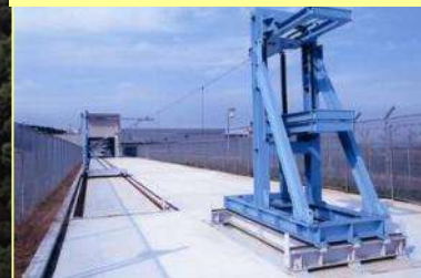
Testing Building B
