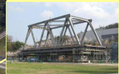
Testing truss bridge
